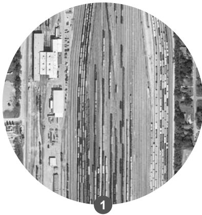
1 Settegast Rail Yard Condition
